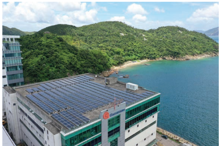
200kWp solar photovoltaic system with sophisticated real-time monitoring to allow for R&D at Gammon Technology Park
